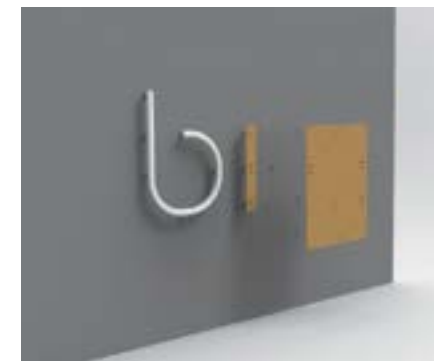
11. Fix letter i on wall pins.
