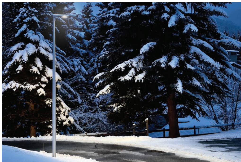
Street lighting - Pontresina, Switzerland Photo: Paolo Carlini
